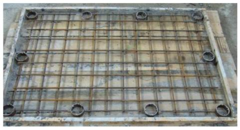
Figure 3. Reinforcement in slabs
