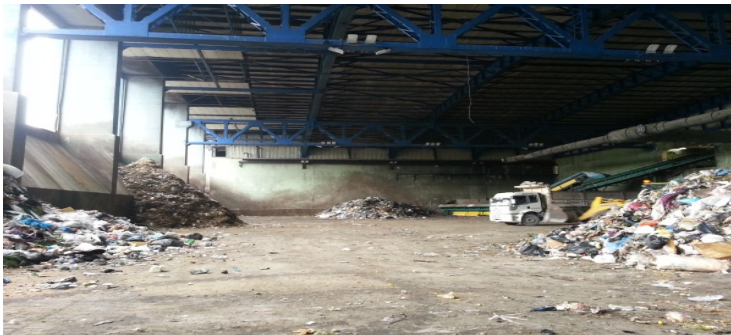
Figure 1. Waste reception unit of the composting plant of IMM
