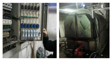
Figure 7. SSR driver table and the controlled heating pump
