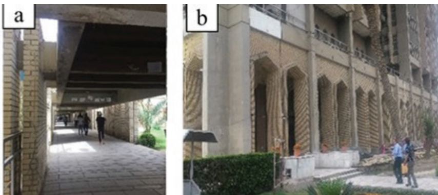
Figure 13. Use of portico. (a) Al-Mustansiriya University. Source: Authors. (b) Baghdad Municipality Building. Source: Authors.
