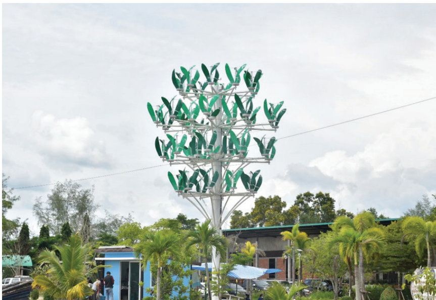
Figure 12. The 15 kW wind turbine pole was installed in Krabi province, Thailand. This wind turbine used the 3 blades with AR=1.5, operating with cut-in at 1.75 m/s that acted under the angles of 120° Twist and 30° Attack.
